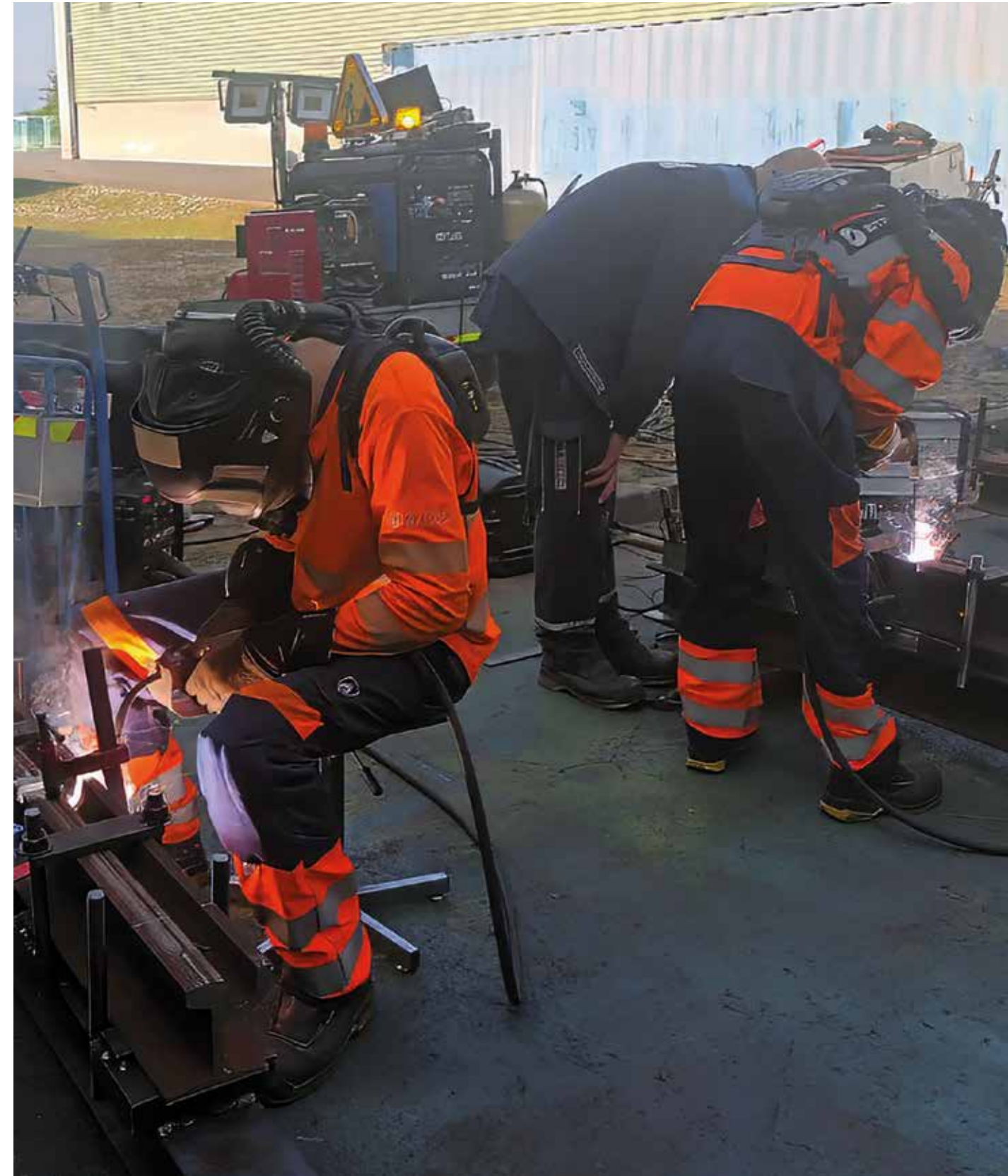
Qualification training for rail butt welding using TRI S RW-0
