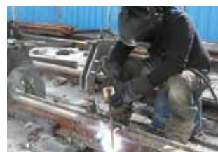
2. Rail butt weld
