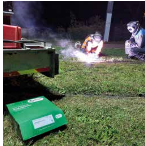
On-site job support to repair a switch section with HARDFACE 19 9 6-0
