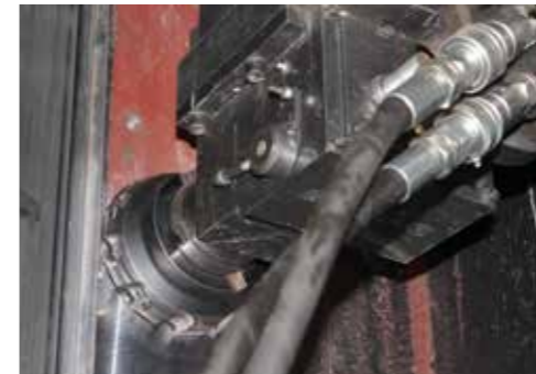
Machining on site.
