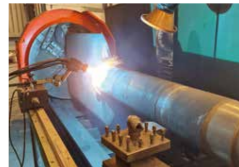
Wire arc spray coating on a wicket gate
