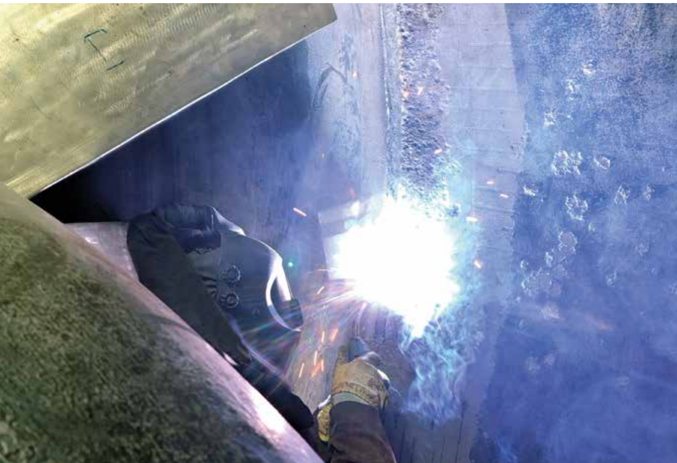
On-site welding repair
